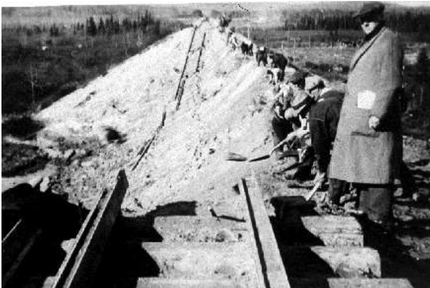
Figure 5: Near Parent, Québec, earthquake vibrations from the 1935 magnitude 6.2 Timiskaming earthquake triggered a 30-metre railway embankment failure, 300 km from the epicentre.
